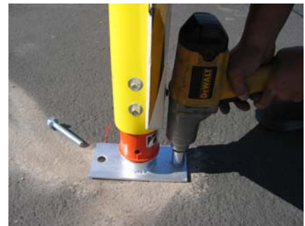
Step 3: Install anchor screws
