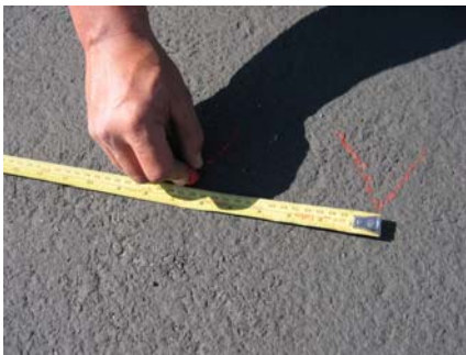
Step 1: Mark hole locations 6-1/2" apart
