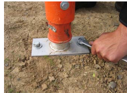
Step 3: Install the post.
