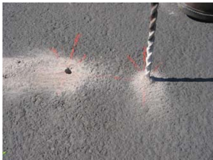
Step 2: Drill holes
